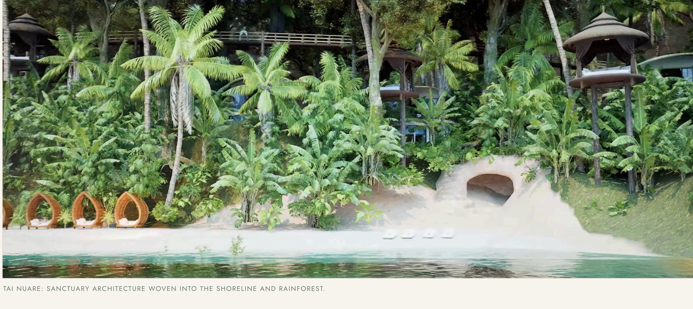
TAI NUARE: SANCTUARY ARCHITECTURE WOVEN INTO THE SHORELINE AND RAINFOREST.
